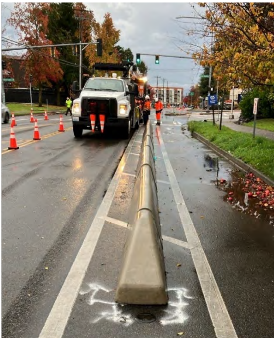
Toronto-style barrier being installed in Seattle
