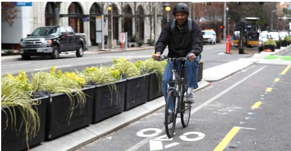
Two-way protected bike lane with planters
