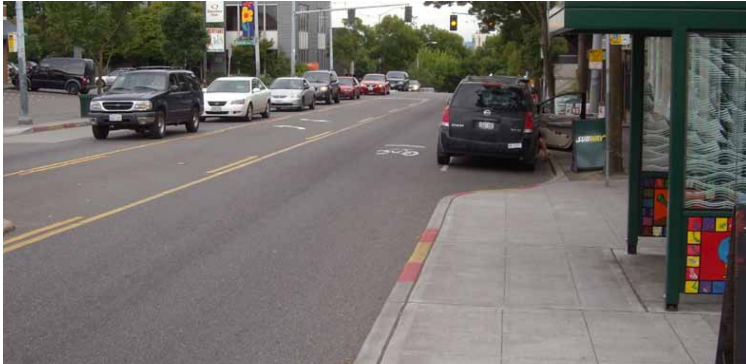
Bus bulbs are a capital improvement that can help meet multiple TMP performance measures: they improve speed/reliability by allowing buses to stop in the travel lane to board passengers and provide additional right-of-way to construct shelters and allow passengers to wait outside of the sidewalk zone.
