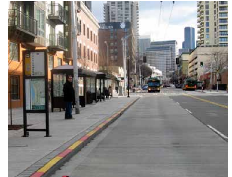
Recent stop improvements along the 3rd Avenue Transit Mall increased stop capacity for passenger queueing and waiting. Image from Seattle DOT
