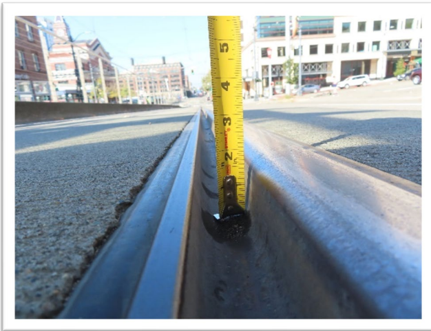
12 Pictured above: Streetcar tracks width and depth shown above exceeds 1.5”, easily trapping bicycle tires.
