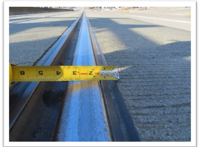
12 Pictured above: Streetcar tracks width and depth shown above exceeds 1.5”, easily trapping bicycle tires.
